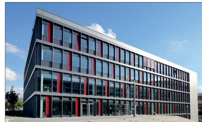
Façade infill panels
