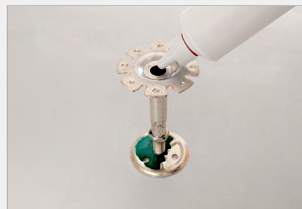
Thread lock of threaded struts
