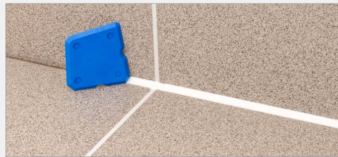
Manual smoothing by means of plastic spatula
